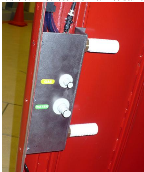
Figure 5.6 – Gondolas outlet sockets for Water and Gas
