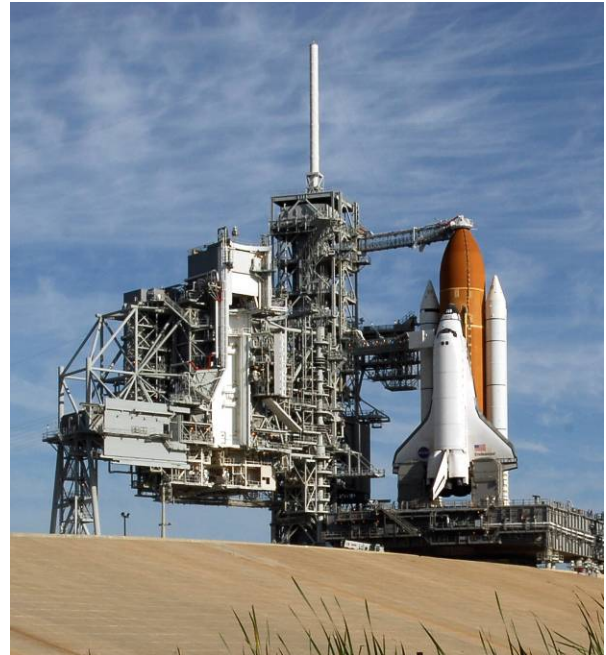
The Rotating Service Structure after rollback to the park position prior to launch of the STS-123 Shuttle Mission on 10 March 2008. (Image: NASA)
