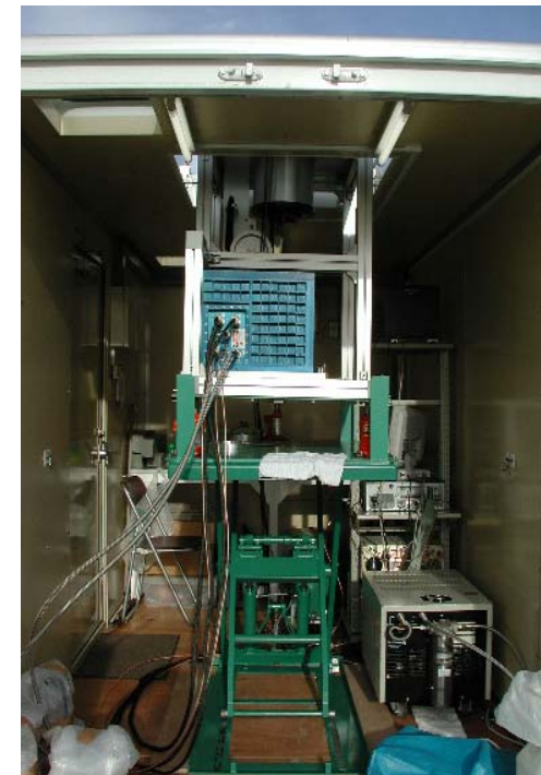
Inside the cargo space with the main body of the lidar colored blue
